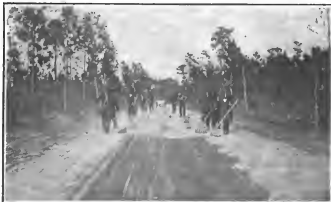
The repair gangs were kept busy right up to the hour of starting
